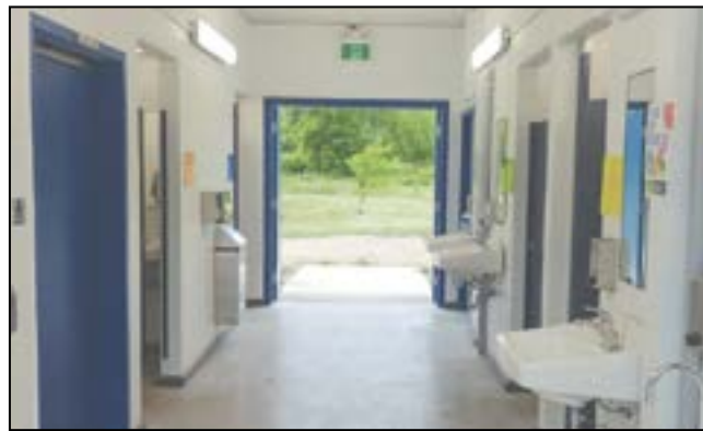
A view through the new bathrooms
